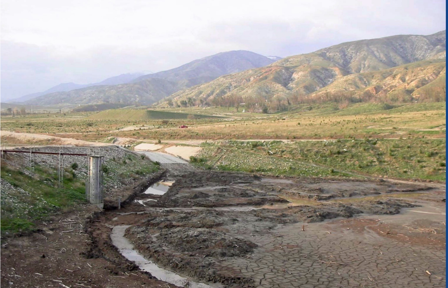
Levee / Photo by SAWPA
