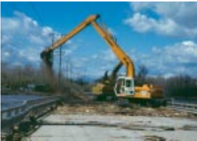
River Road Bridge, 1998
